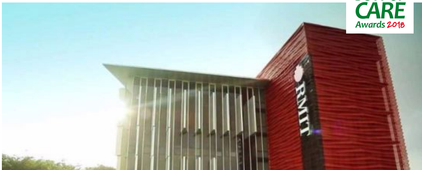
Above: RMIT Vietnam's State of the Art Academic Building.
